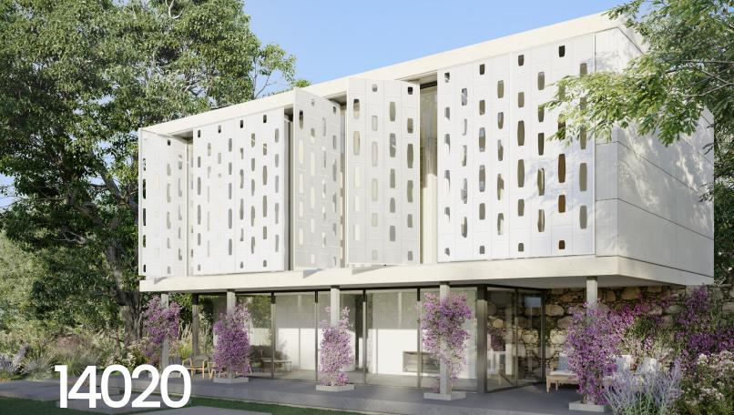
Kinetic Façade Horizontal Independent Pivot Shading System
