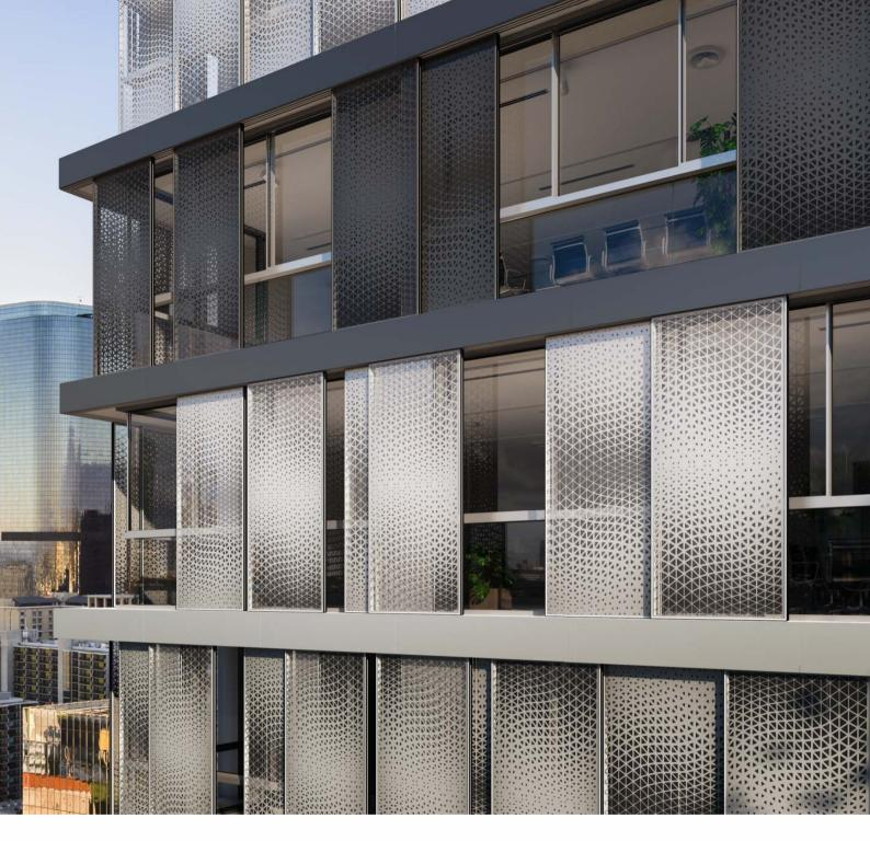
The system has been designed to allow for seamless integration with the building external cladding. Several versions are available to be used with fiber cement, HPL, Aluminium composite panels, wood, glass, ceramic and metal sheets. Provision has been taken to allow the use of cladding material on the shading system itself. In addition to the cladding material, the system comes with a variety of blades to be installed vertically or horizontally.
